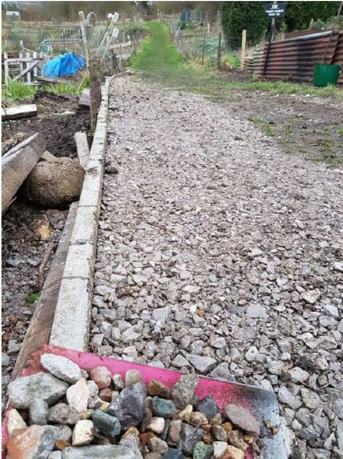
Roadworks on Sunnyside New
